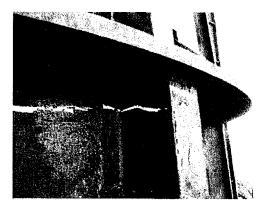
The shell crack migrates to the upper weld of the ring stiffener at the North-west vertical stiffener.
