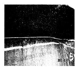
At the South-west vertical stiffener on the top side of the ring stiffener plate the shell is cracked approximately twenty-four (24) inches.
