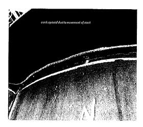
The shell crack continues through the web section and connection welds of the North-west stiffener.
