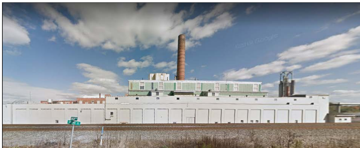
Morton Salt plant in Silver Springs, New York
