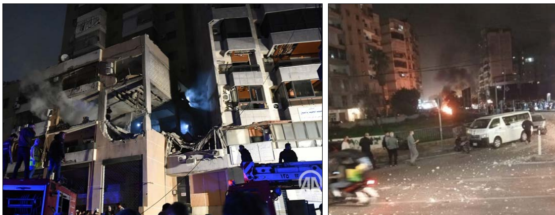
Building in Dahieh, the southern suburb of Beirut, Lebanon where al-Arouri was killed.
