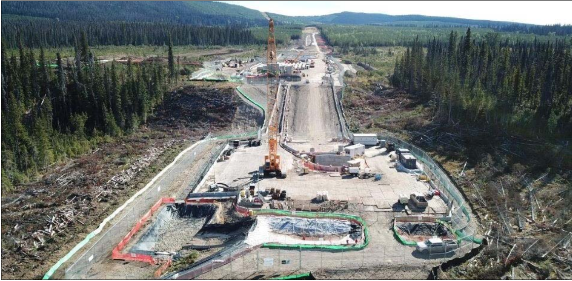
Drill pad constructed by Coastal GasLink to drill under Wedzin Kwa headwaters, September 18, 2022
