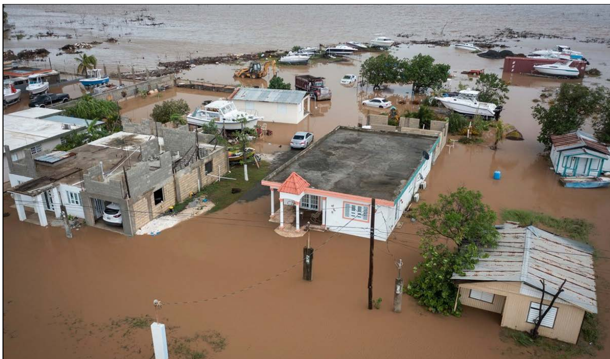
Devastation caused by hurricane Fiona in Puerto Rico, September 2022
