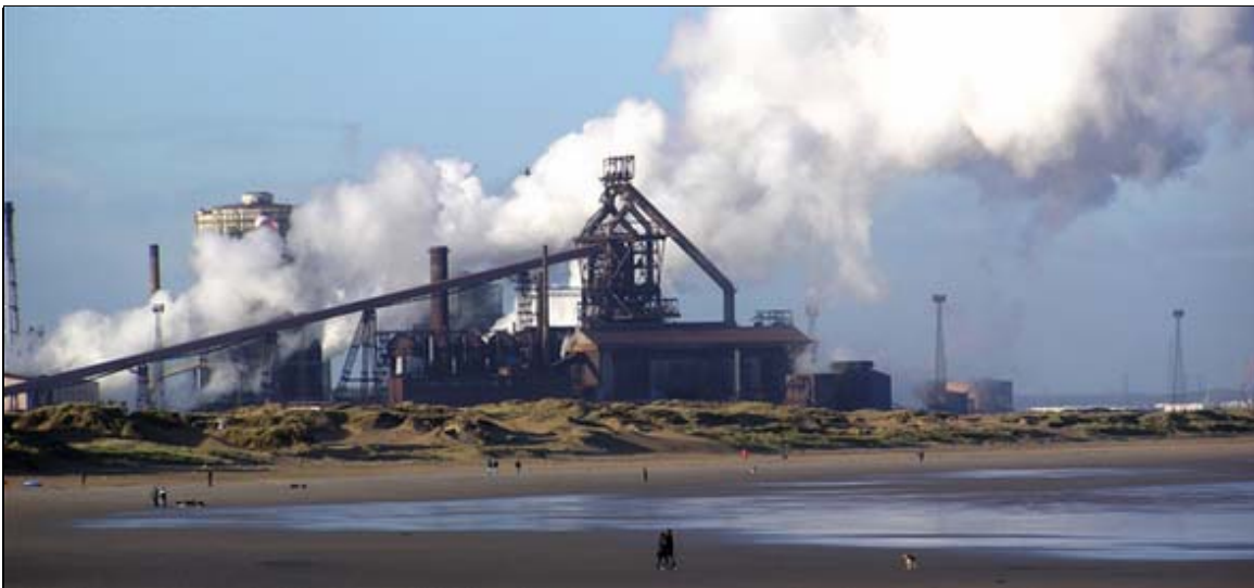
Redcar steel works prior its closure in 2015
