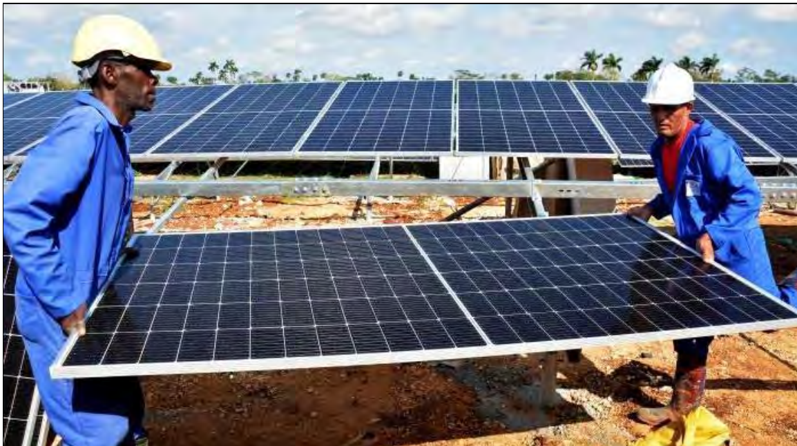
Installing solar panels in Villa Clara in Sanctis Spiritus, January 2026
