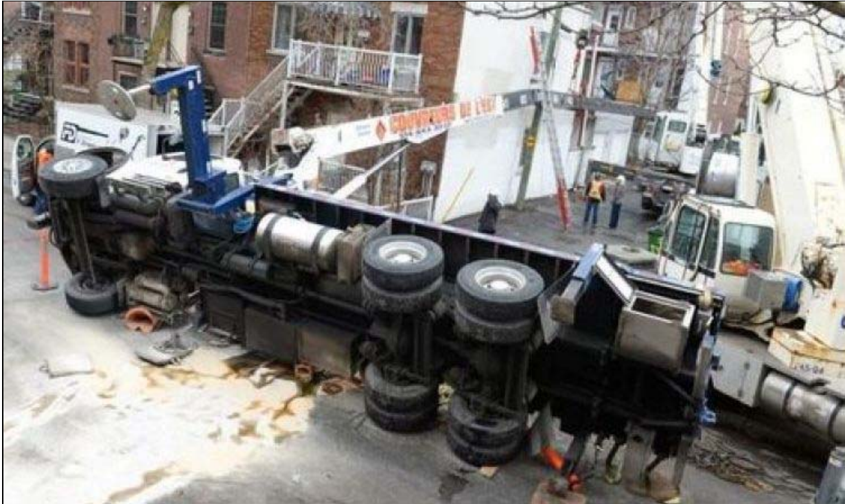
Picture of overturned boom truck in Montreal, April 19, 2018, posted to crane operators facebook page.
